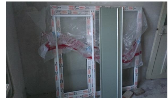
Working on putting in new windows
